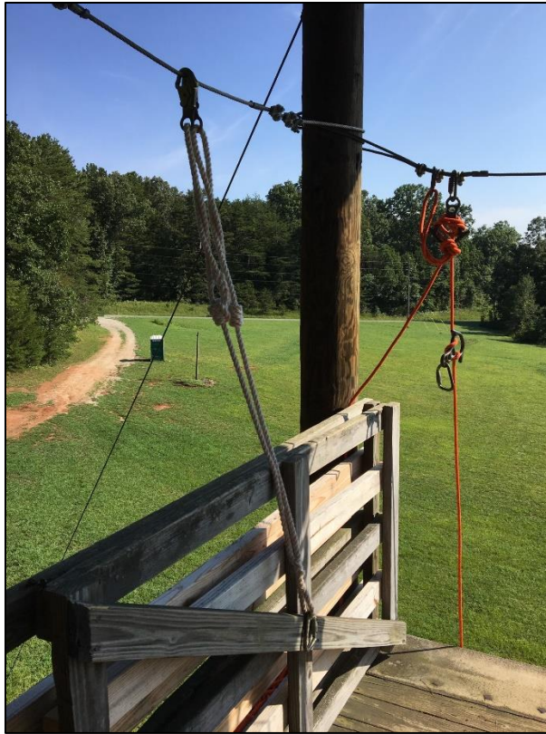
The rappel platform at MSR showing the participant tether on the left and the rappel line in orange.
