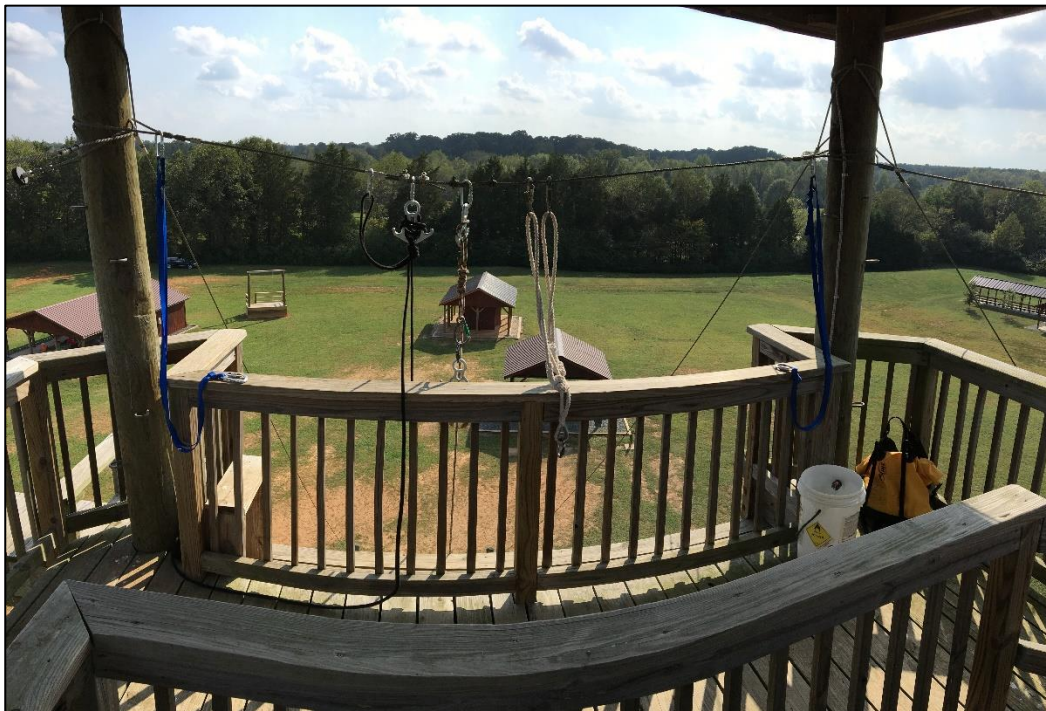
Complete rappel rigging at Belk including all tethers.
