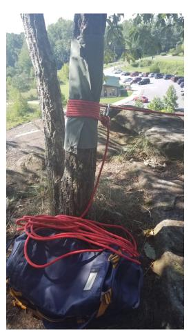
Once at these trees, protect the larger tree with a canvas pad, then make a single wrap around the tree with the rope. Then pull on the rope to apply tension to the tether system. Once the rope has been tensioned, continue wrapping the tree with the rope to create a tensionless wrap with a minimum of 4 wraps.
