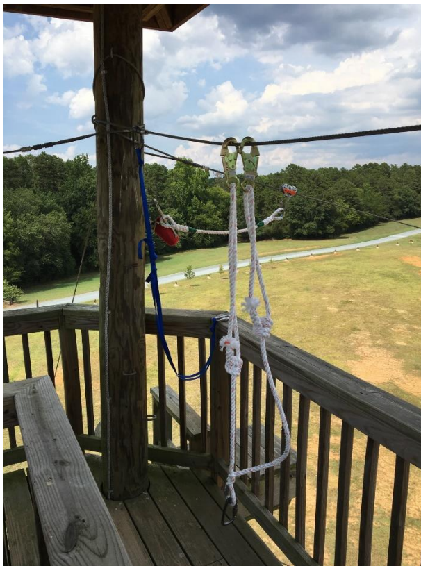
Completed zip line rigging at Belk.
