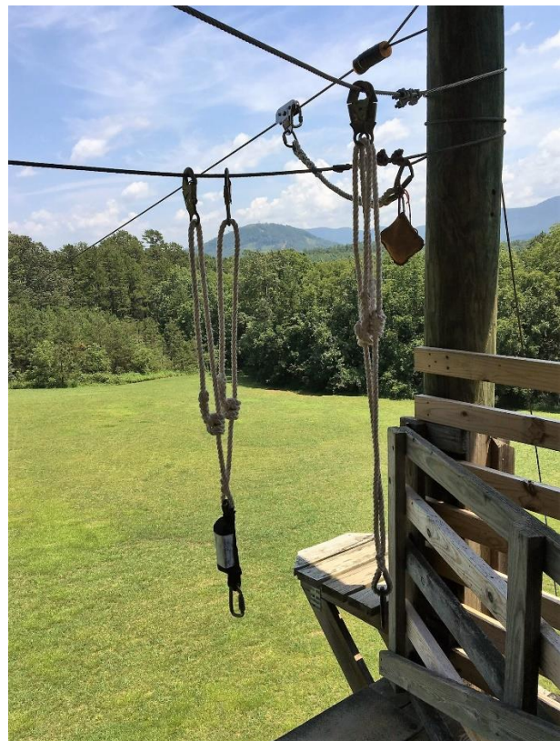
Completed zip line rigging at MSR. Note the participant tether is a set of lobster claws without the Zorber.
